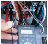
If the DC voltage between communication terminal A, B of indoor unit fluctuates within -9V ~ +9V, then the communication from the outdoor unit is normal.
